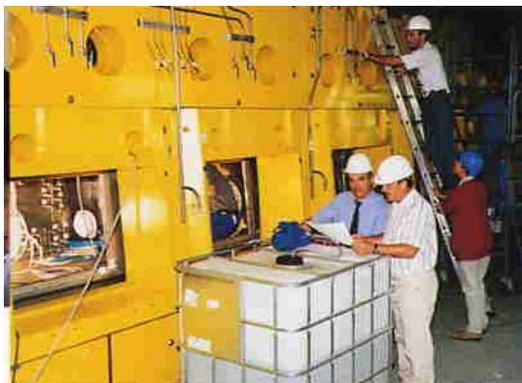
Together with the CEA, SGN is building Atalante DRA, the new research laboratory on the back end of the fuel cycle, at the Marcoule site. Here, installation of shielded analytical lines.
